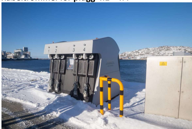
Kabeltrommel for plugg 4.1 - 4.4
